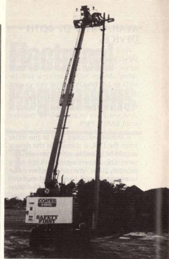
Coates JLG both boom onsite at Blue Circle Cement's, Berrima Works.
